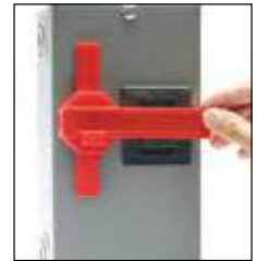
Slide Stop Bar into position over breaker
