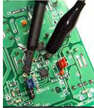
Fig. 4C Connecting O-scope probe to hook Gate drive test points.
