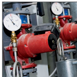
Sensors, valves and control cabinets
