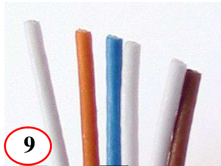
9 Trim ends of Org Blu and Brn pairs @ slight angle to make loading easier
