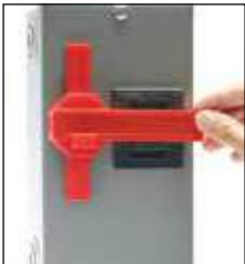
Slide Stop Bar into position over breaker
